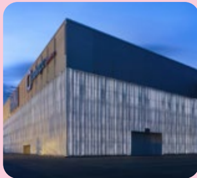
↑ Palexpo Palexpo offers 106,000 m 2 of pillar-free multi-functional areas all under a single roof, including a convention centre seating from 100 to 2,500 participants. → Palexpo
